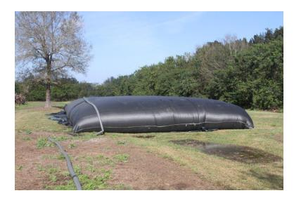
• Once dewatering is completed (up to 3 months), sediments from geotextile bags will be treated for Acid Sulfate Soils and transported to the Vidler Road Waste Facility in Dunsborough for reuse.
