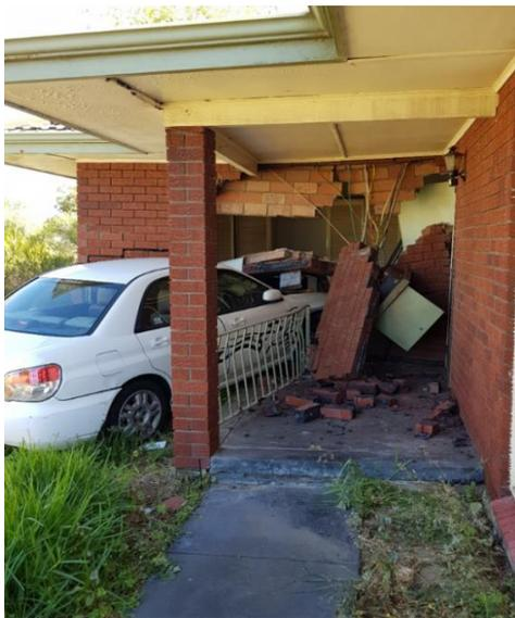
A reconnaissance of the building was conducted by the SES crews, with the attached photograph indicating the scene upon arrival. Western Power stickers were identified inside the main meter box, indicating that power had been isolated due to pending demolition, but there was no labelling noted to point to the presence of an Alternative Energy System (AES).
