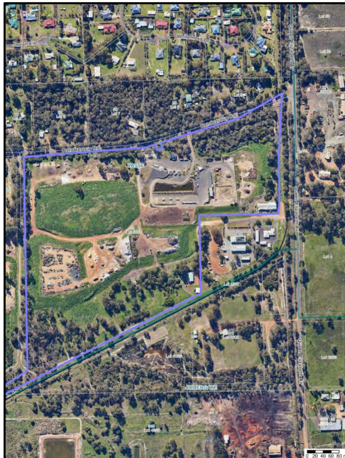
Figure 1: Busselton Waste Transfer & Recycling Centre (BWTRC), Lot 500, 39 Rendezvous Rd Vasse.
