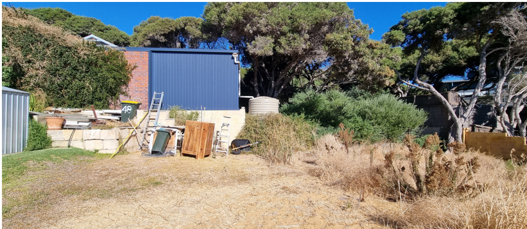
Photo 4 : Taken from the centre of the Site facing south
