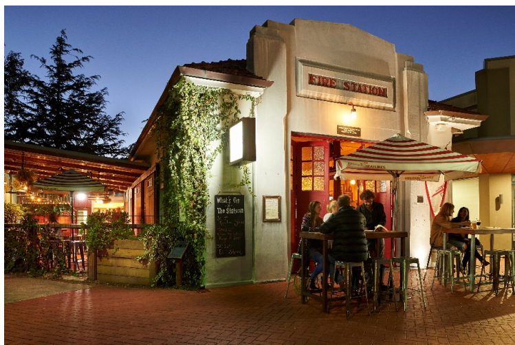
Above – 5.3.3.c : Busselton Fire Station No. 2 (former) – example of later addition not obscuring elements of Cultural Heritage Significance.
