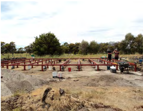
Restumping the Hall, 2014. Courtesy current owners.
