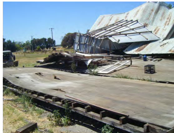
Collapse after storm, 2013. Courtesy current owners.
