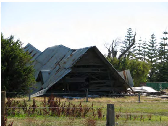
Collapse after storm, 2013. Courtesy current owners.
