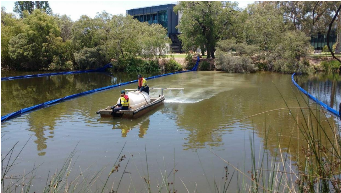
Figure 18. HT clay being applied in the Lower Vasse River during the 2017-18 trial.
