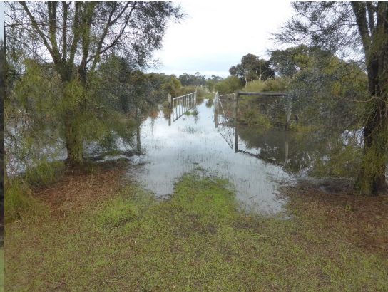
Figure 3-14 Foot bridge (WP 2)
