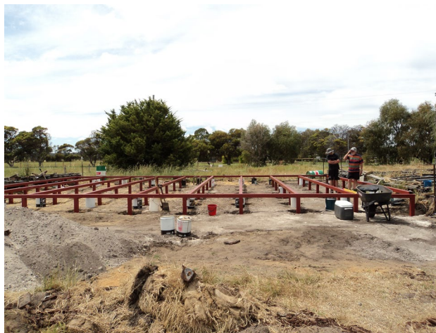
Restumping the Hall, 2014. Courtesy current owners.
