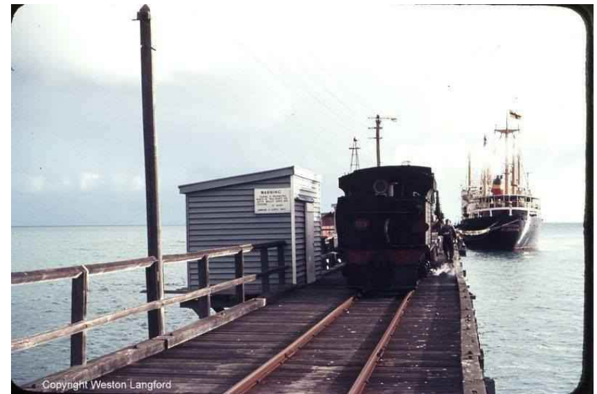
Image 25: Steam locomotive on Busselton Jetty c1960s. Note the traditional balustrade and kerb rail details and the utilitarian style of the building projecting off the jetty neck. Busselton Heritage Trail online gallery image 14-6, noted as Copyright Weston Langford.
