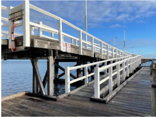
Photo 33: View of access ramp to lower platform 2A. H+H Architects, 2022.
