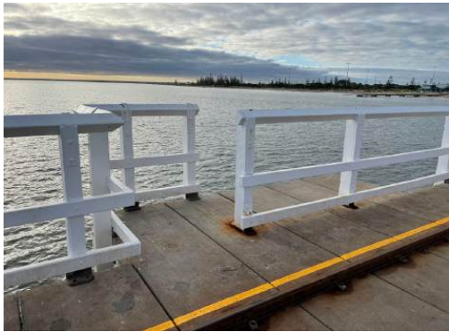
Photo 23: Detail view of upper landing, Section 2, Busselton Jetty. H+H Architects, 2022.
