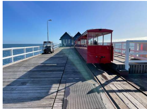
Photo 60: View of Gerry Bovell Platform, Section 7, Busselton Jetty. H+H Architects, 2022.
