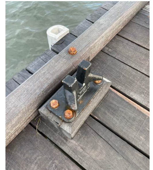
Photo 32: Detail view of mooring bollard to lower platform. H+H Architects, 2022.
