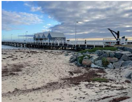
Photo 8: View of landing of Busselton Jetty showing groyne and beach setting. H+H Architects, 2022.
