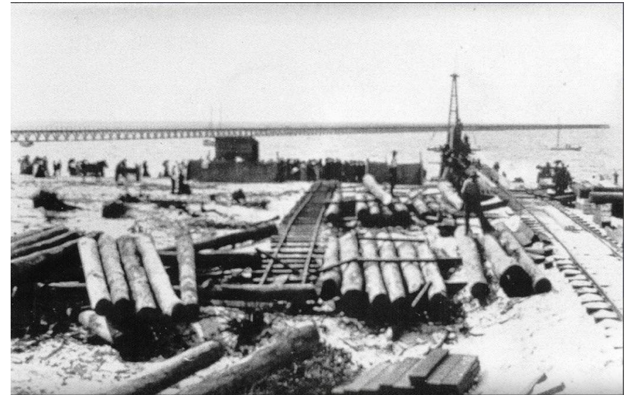
Image 10: Building the Skeleton Jetty 1909, note the rail line extending from the Stanley Street alignment to join up with the main jetty. Busselton Heritage Trail online gallery image 26-7.
