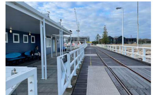
Photo 18: View of Jetty Section 1- East and Section 1- West. H+H Architects, 2022.
