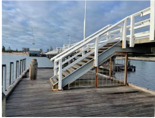
Photo 34: View of access stair to lower platform 2A. H+H Architects, 2022.
