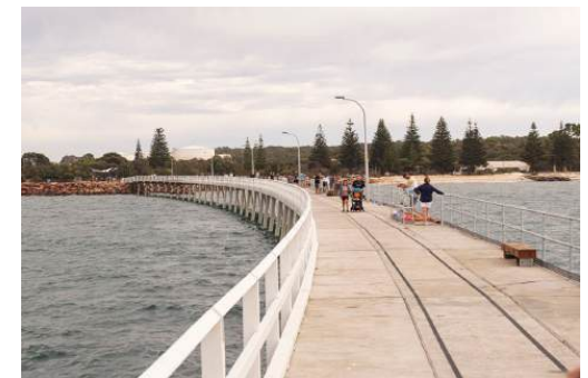
Photo 77: View of concrete deck to majority of Replacement Esperance Jetty. H+H Architects, 2022.
