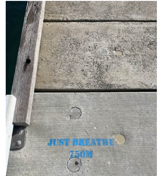
Photo 44: Detail view of concrete panels showing different finish between Jetty Sections 3 and 4. H+H Architects, 2022.
