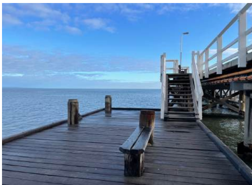
Photo 27: Detail view of Platform 2B, Section 2, Busselton Jetty. H+H Architects, 2022.
