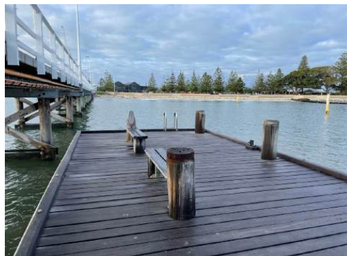
Photo 28: Detail view of Platform 2B, Section 2, Busselton Jetty. H+H Architects, 2022.
