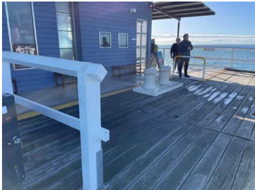
Photo 59: Pair of mooring bollards located near terminus of tourist tram and Underwater Observatory, Section 7, Busselton Jetty. H+H Architects, 2022.
