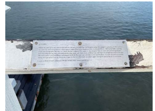
Photo 6: Detail view of typical interpretive panel at Busselton Jetty. H+H Architects, 2022.
