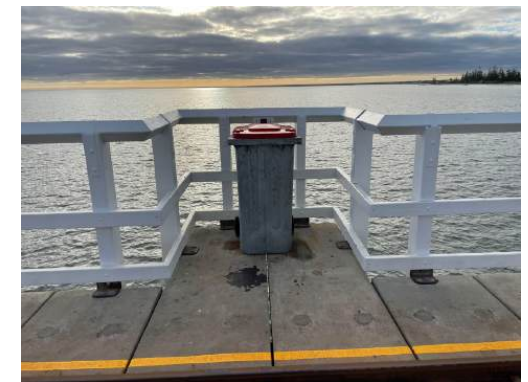
Photo 7: Detail view of typical bin recess at Busselton Jetty. H+H Architects, 2022.
