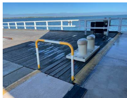
Photo 65: Pair of mooring bollards located near terminus of tourist tram and Underwater Observatory, Busselton Jetty. H+H Architects, 2022.
