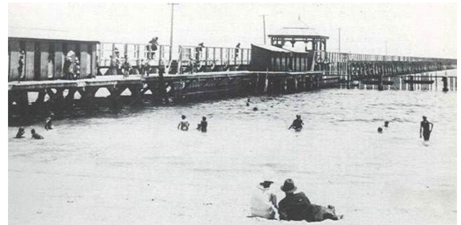
Image 15: Photograph of Busselton Jetty c1920s. Battye Library Pictorial Collection, 25406P.
