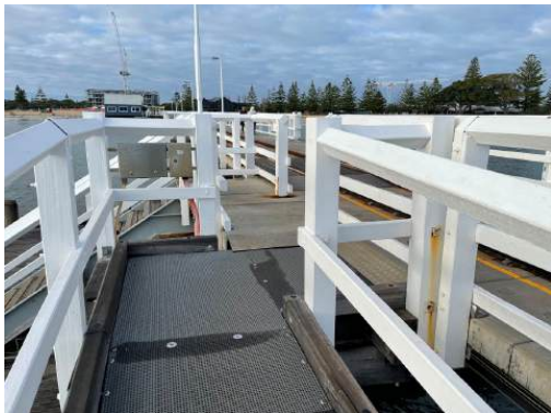
Photo 37: View of upper landing to lower platform 2A. H+H Architects, 2022.
