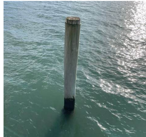
Photo 43: View of free-standing pile in Section 3, Busselton Jetty. H+H Architects, 2022.
