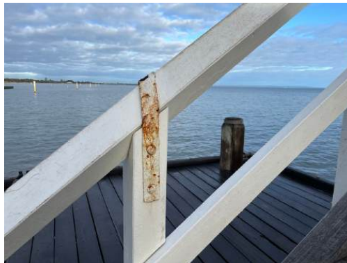
Photo 38: Detail view of strapping to top rail of balustrade. H+H Architects, 2022.
