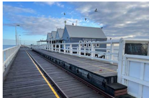
Photo 16: View of Roy Morris Platform in Jetty Section 1- West. H+H Architects, 2022.
