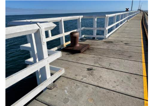
Photo 50: View of salvaged mooring bollard, Jetty Section 5, Busselton Jetty. H+H Architects, 2022.
