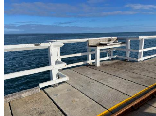
Photo 49: View of fish cleaning station, Section 5, Busselton Jetty. H+H Architects, 2022.
