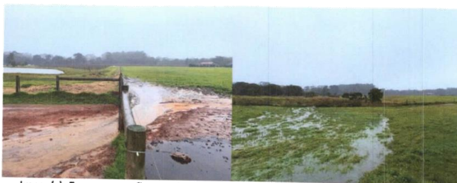
Image(s): Excess water flowing from Lot 100 onto neighbouring properties 852 + 853
