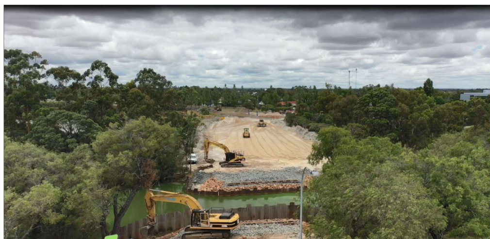
Photo: Eastern Link Works In Progress 5
