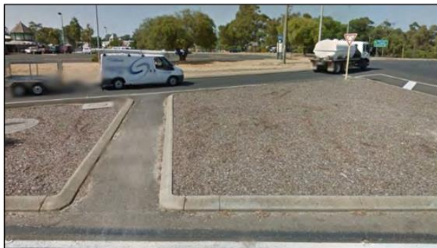
Poor pedestrian/cyclist access to the TC from Dunsborough Playing Fields
