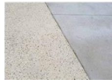
PAVING - IN-SITU POURED CONCRETE
