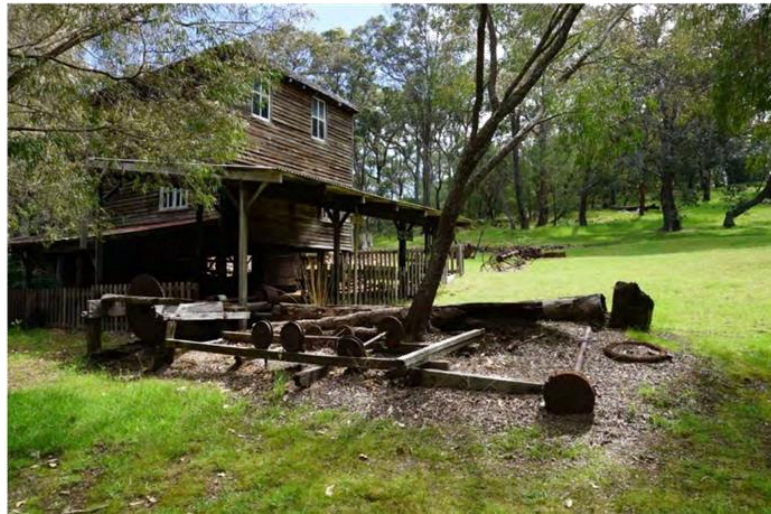
Plate 2: Millbrook Mill and maintained grounds, looking west towards the building.
