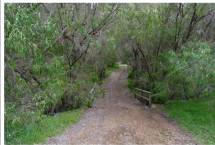
Photo location 24: existing fire services access route/emergency access way within the southern portion of the site.
