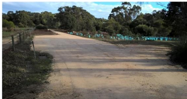
Limestone sheeting works at the corner of the Wildlife Corridor and Western firebreak
