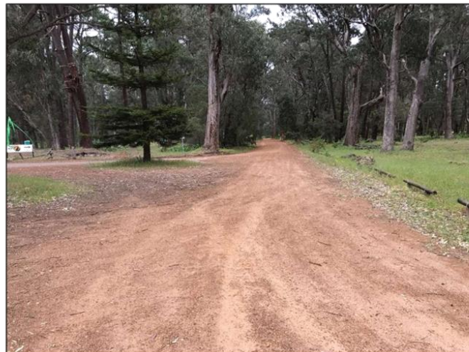
Finding 2.1.2 – The Ludlow Park Road intersection forms a Y junction. This can lead to confusion among drivers. The gravel section should be removed or barricaded from vehicles.
