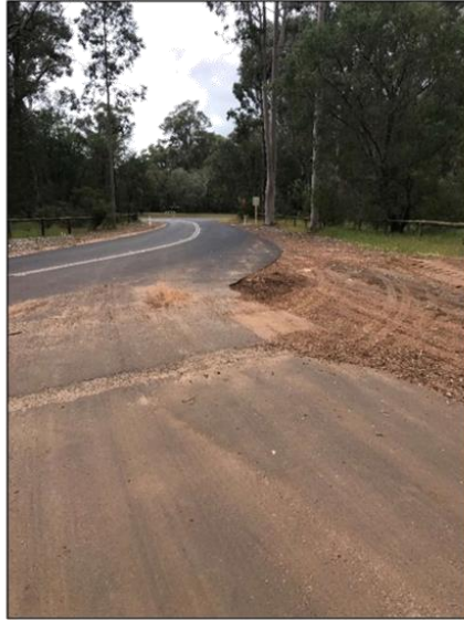
Finding 2.2.1 – Drivers are shortcutting onto the gravel edge and spreading loose material onto the intersection.
