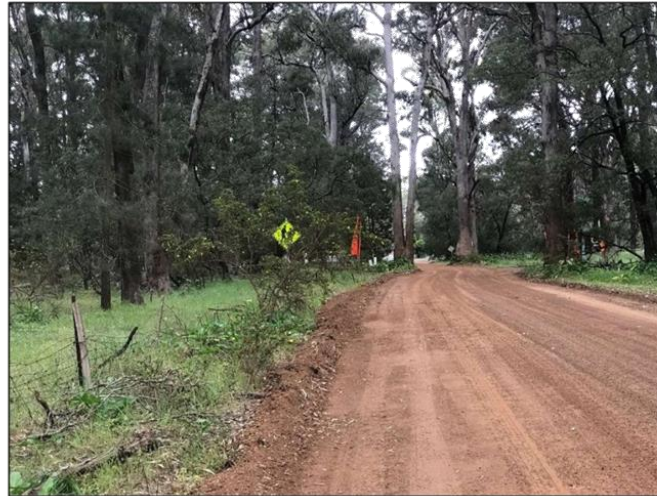
Finding 2.1.3 – The vegetation partly obscures the advance warning sign of the pedestrian crossing eastbound.
