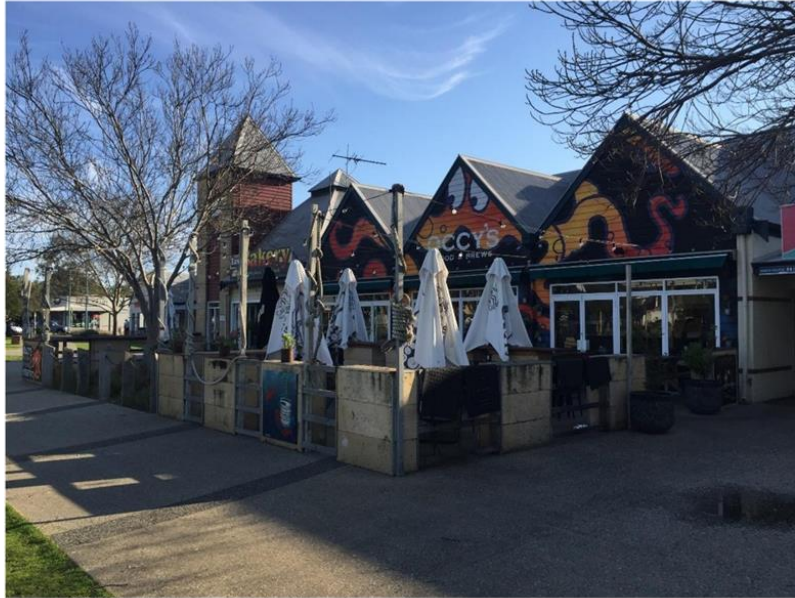
Existing Development – Lot 1 (12/34) Dunn Bay Road, Dunsborough
