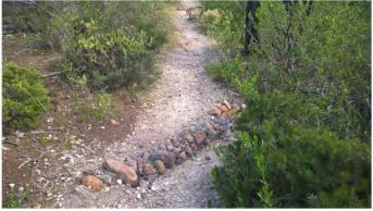
Rock riffle installed to prevent trail soil erosion
