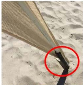
Star picket deep in sand, two cable ties holding leg to star picket
