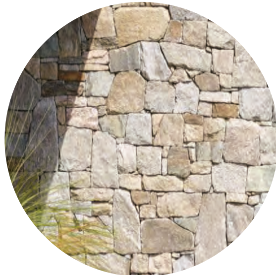
NATURAL STONE CLADDING TO WALLS
