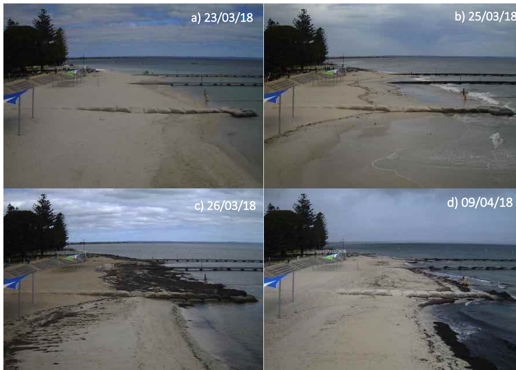
Figure 4.6 Busselton Jetty Fixed Camera Monitoring showing wave runup (b) and wrack deposition associated with TC Marcos (c) and localised scour downdrift of groyne (d)
