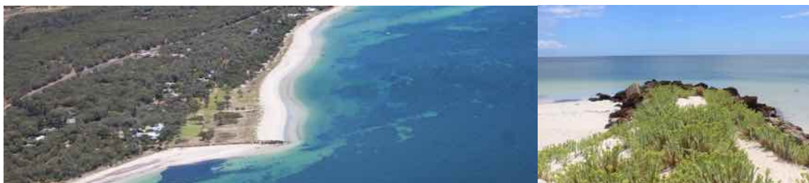
Figure 7.3 Siesta Park Groyne (Dec 2017)
