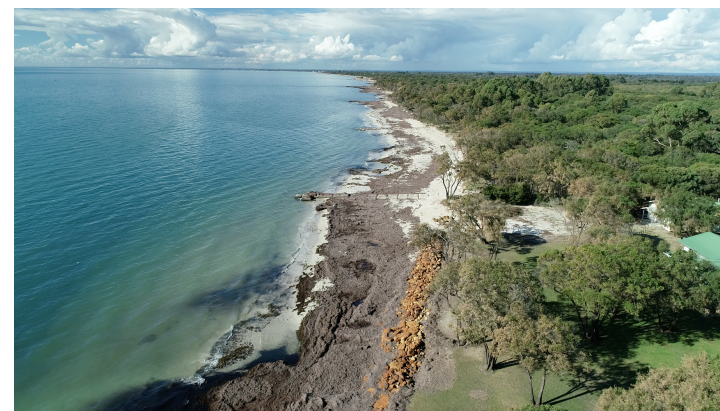
Figure 2.9 Screenshot of UAV drone footage (Locke Estate)
