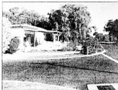
Figure 13: Cafe on North Street
