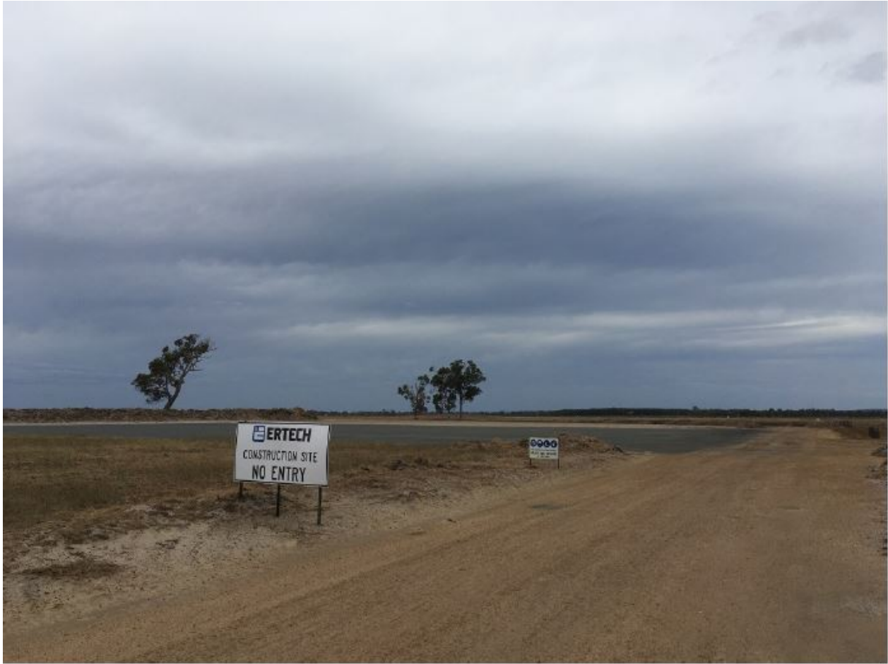
Batching plant site preparation
