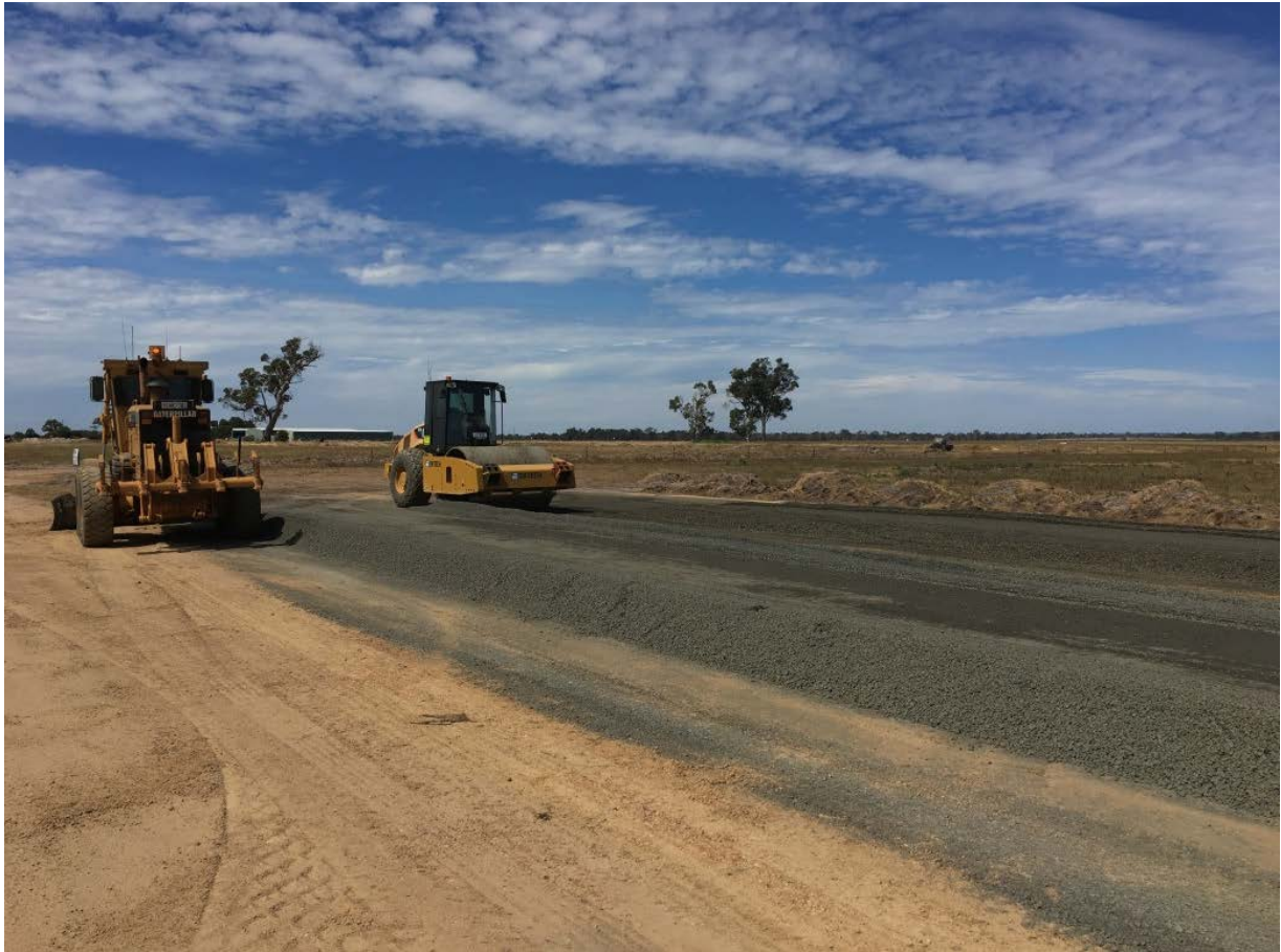
Pavement testing area
