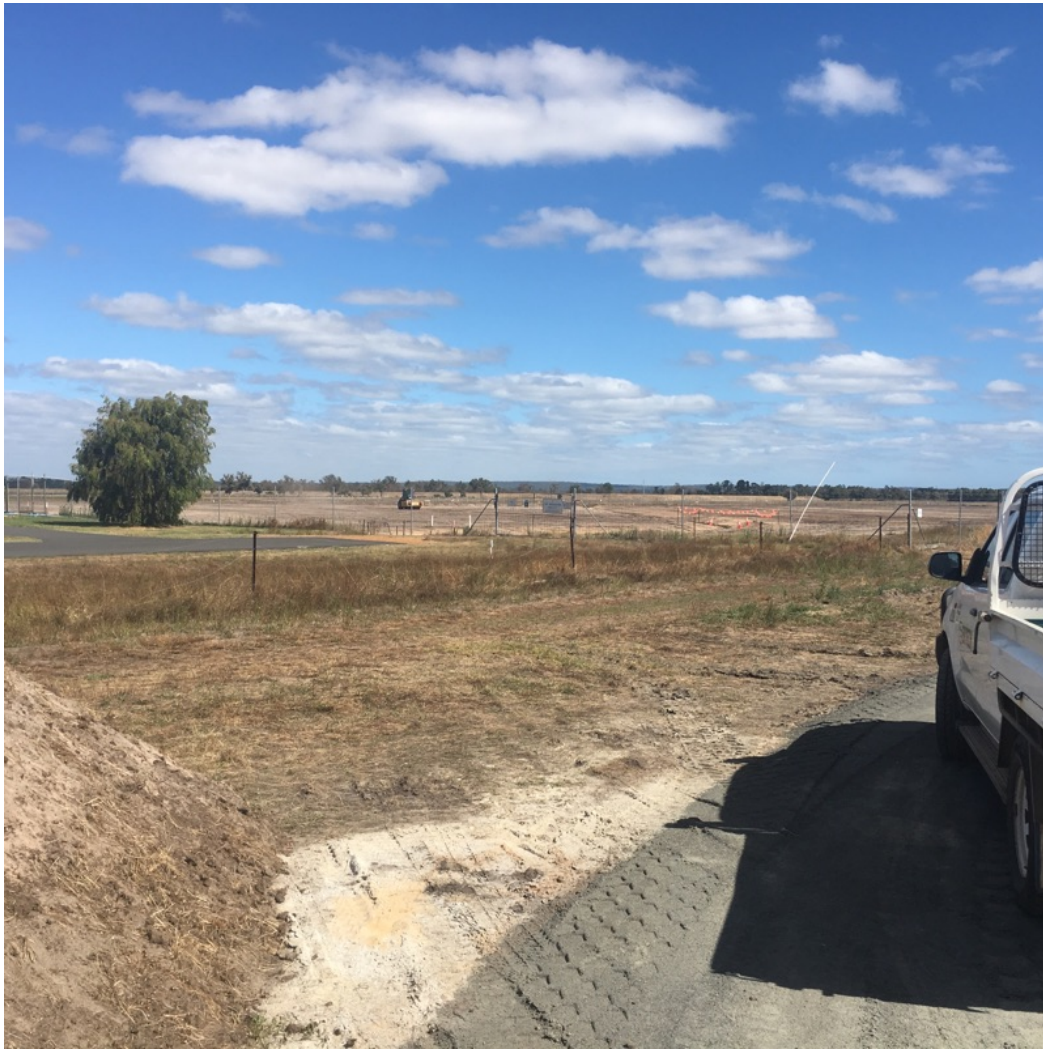
Looking out to new apron: site preparation works underway
