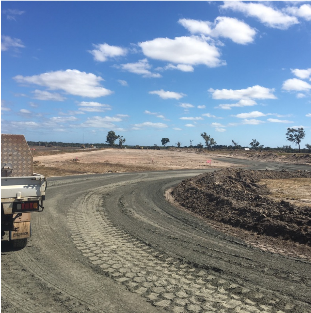
Internal construction roads
