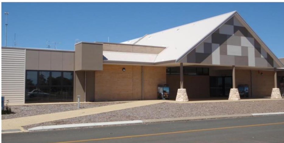
Figure 14 Passenger terminal building
