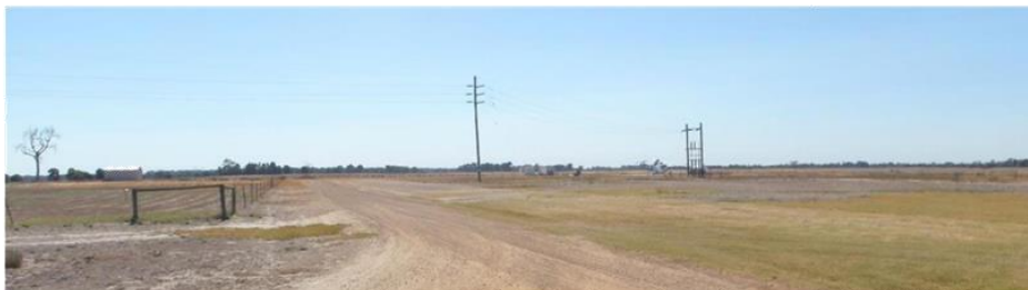
Figure 17 Overhead transmission lines go underground to the north of the current terminal
