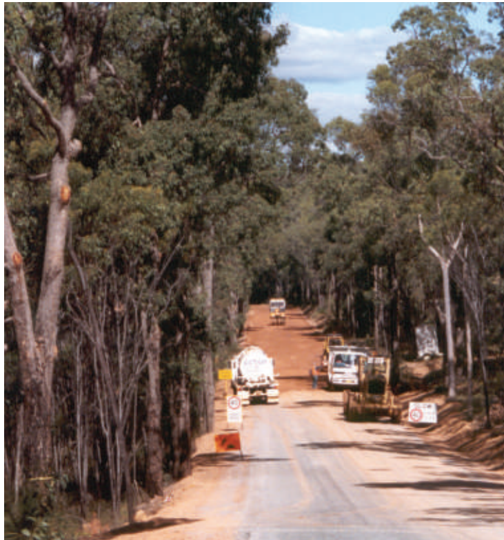
Road construction with Phytophthora Dieback infected soil or gravel can lead to the introduction of the disease to adjacent bushland.
